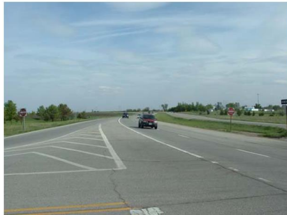
Offset Right Turn Lane Source: Review of Iowa's Rural Intersection Crashes: Application of Methodology for Identifying Intersections for IDS (MnDOT, MN/RC 2007-27)
